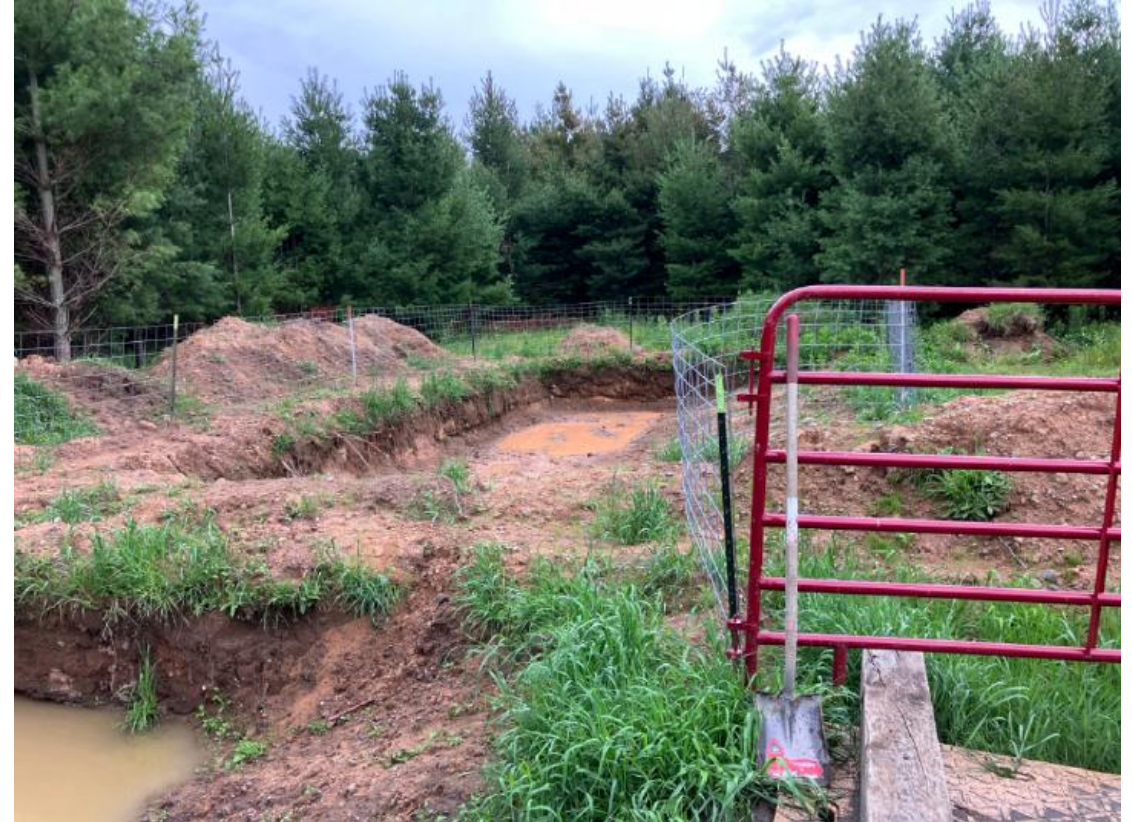
Talon sump adjacent to mats over wetlands (Source: DNR 2024-08-07 right)
