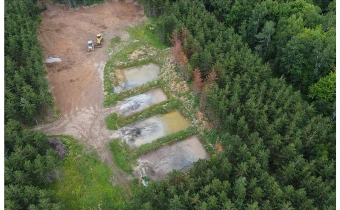
RIO TINTO - TALON METALS HEADQUARTERS | DRILLING FLUID SUMPS
