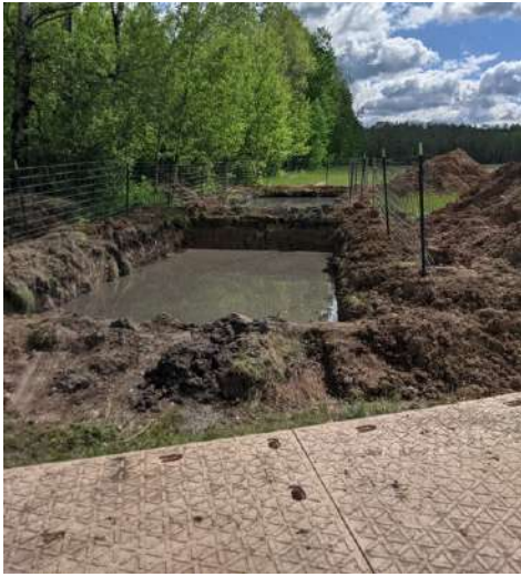
Unlined sump in wetlands, swamp mats (DNR 2022)
